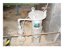
**c.** Open Valve after Bag Filter to the Inlet Port on the SEPARADE-R.
